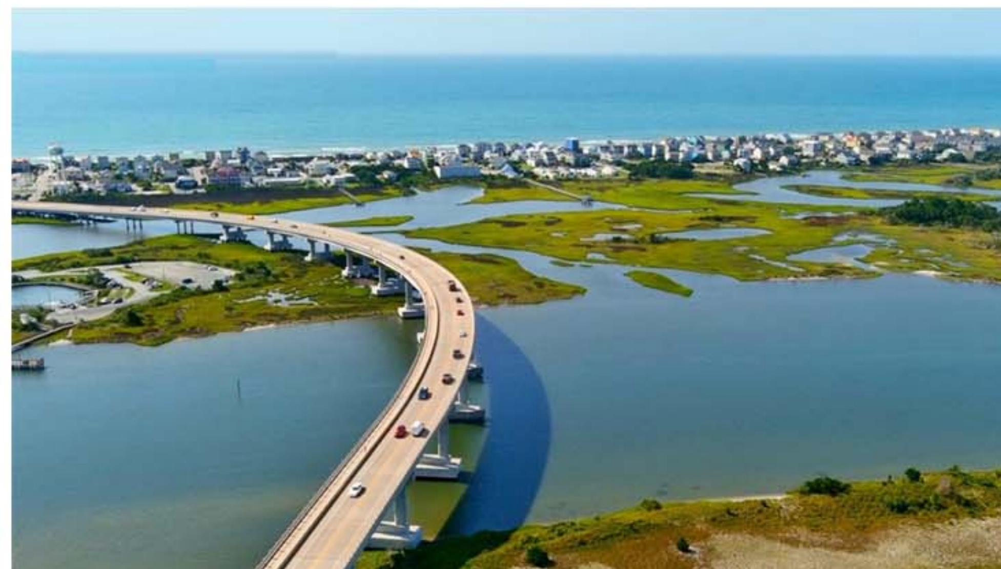
Surf City Expansion Bridge
